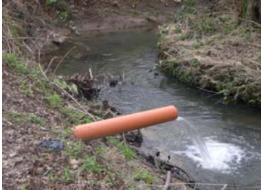
The new outlet to the stream
