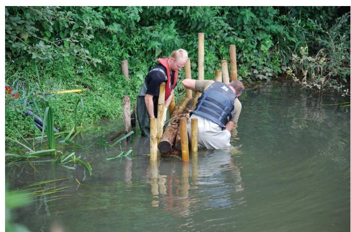
Wiring the woody sections to the posts
