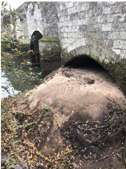
Sediment build up at Fittleworth Bridge
